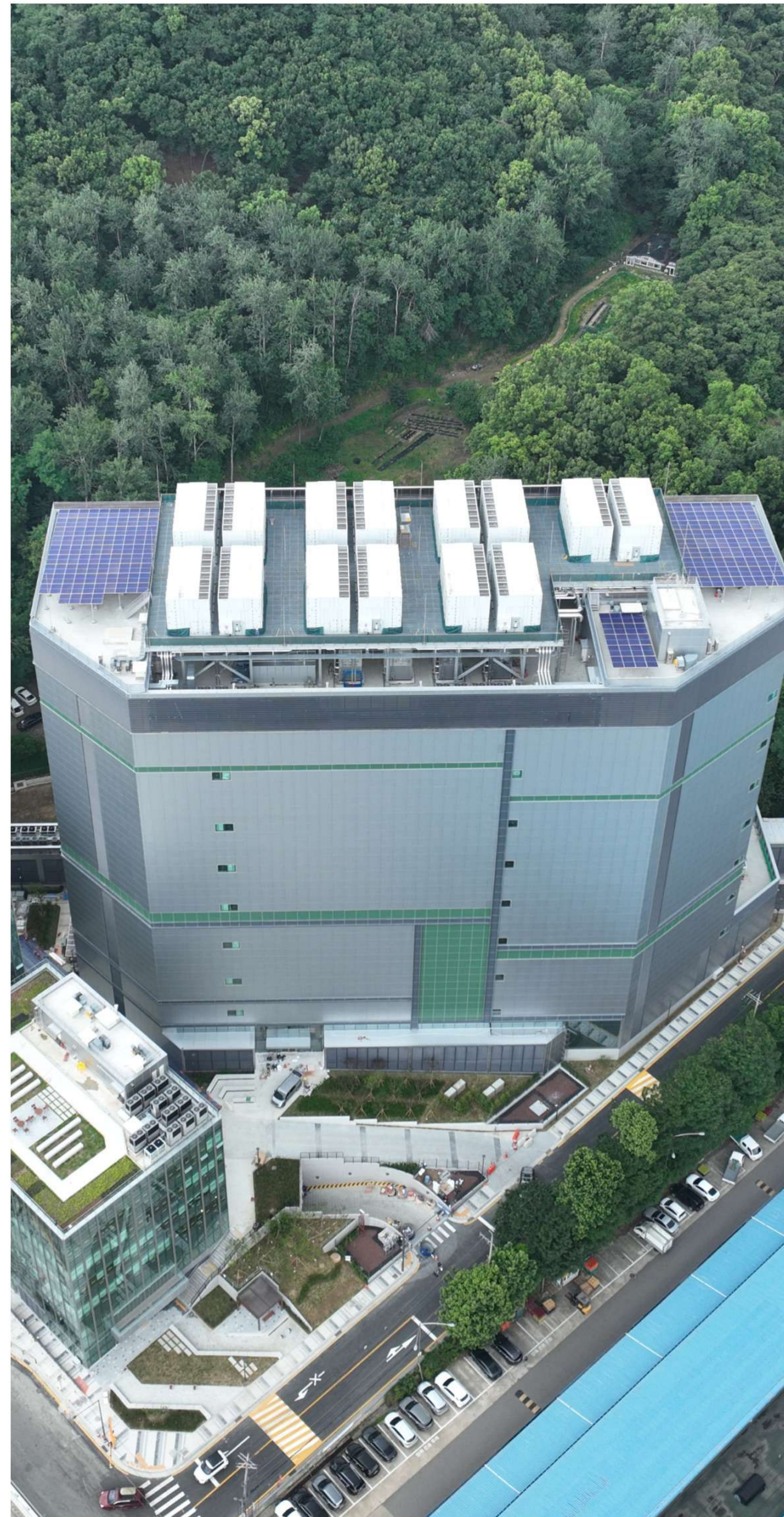
Integration of rooftop solar and building-integrated photovoltaics at Empyrion Digital's KR1 Gangnam Data Centre campus, South Korea
